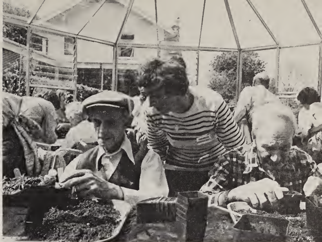
A view from outside of a general activity class in the octagonal Horticultural Therapy Greenhouse. Note the absence of a central support, and the way in which wheelchairs can be drawn up to the benches. Photo: Sylvia Taylor
